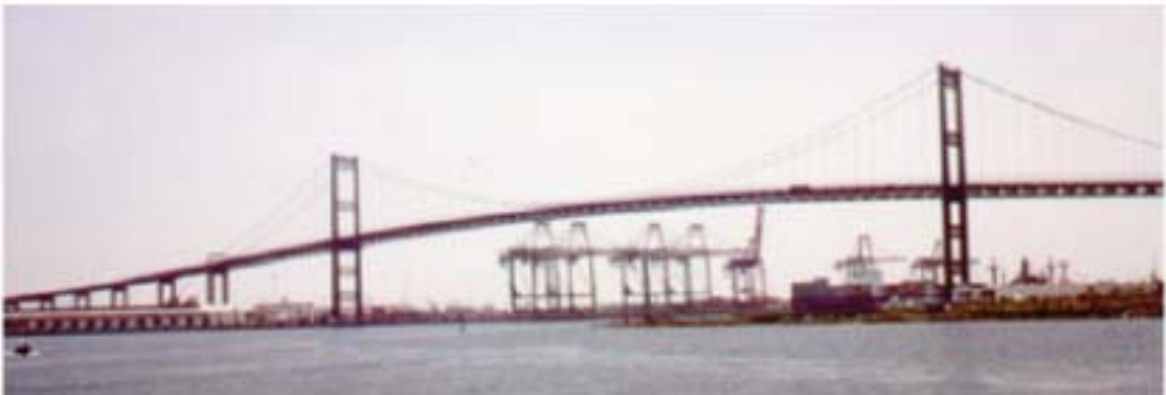
FIGURE 30.87 The Vincent Thomas Bridge, a three-span suspension structure built over the Port of Los Angeles.
