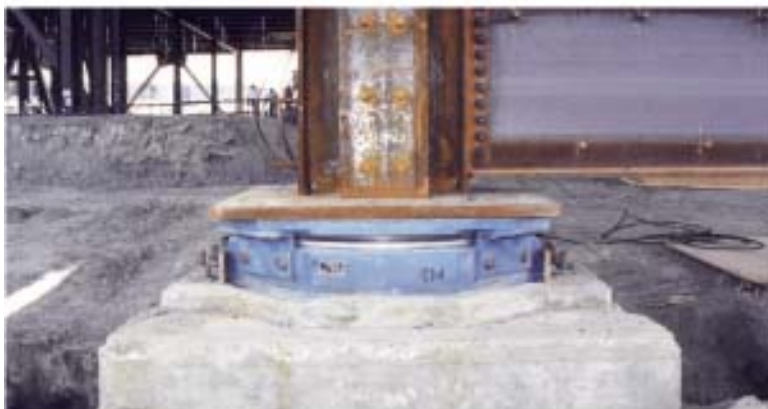
FIGURE 30.79 One of the 267 friction pendulum devices for the new San Francisco Airport International Terminal. (Courtesy of Earthquake Protection Systems, Inc.)
