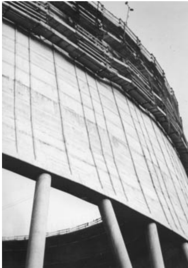
FIGURE 14.40: Column to lintel connection.
