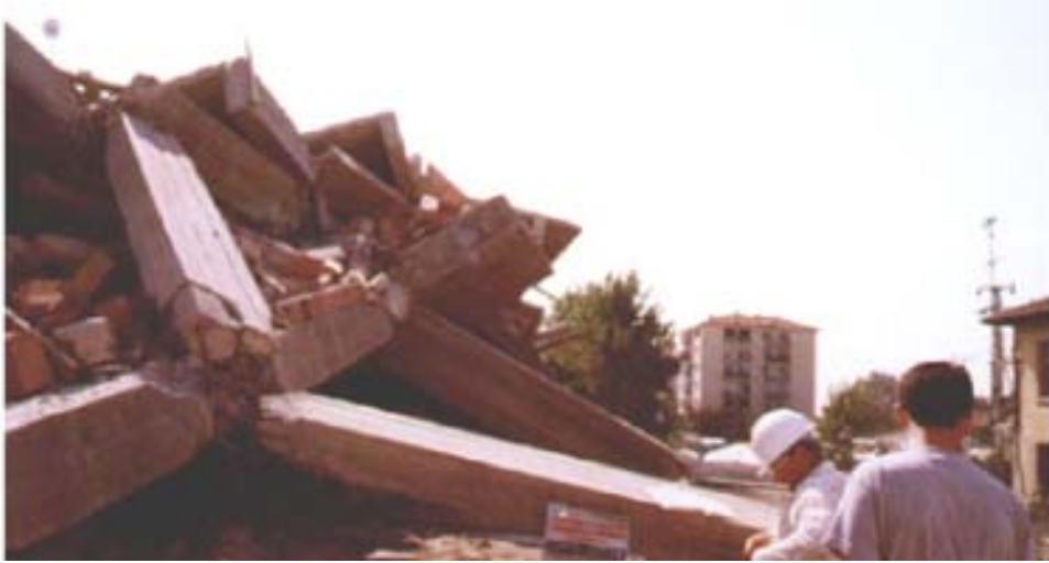
FIGURE 30.59 Collapsed reinforced-concrete building during the 1999 Kocaeli earthquake.
