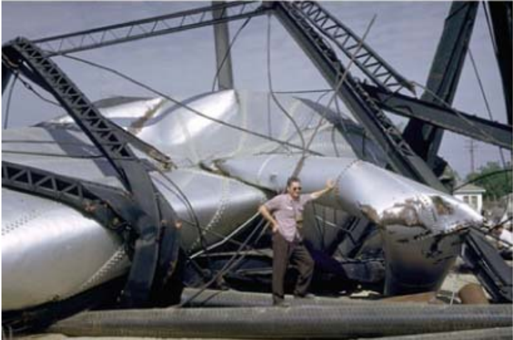
FIGURE 30.62 California Water Service 150,000-gallon tank on six legs (Bakersfield, CA). The typical failure of tanks is upside down, with riser on top. Photograph taken July 25, 1952, after the July 21, 1952, Kern County, CA earthquake (magnitude 7.69). (Photograph by Karl Steinbrugge and courtesy of the Steinbrugge Collection, Earthquake Engineering Research Center, University of California, Berkeley.)
