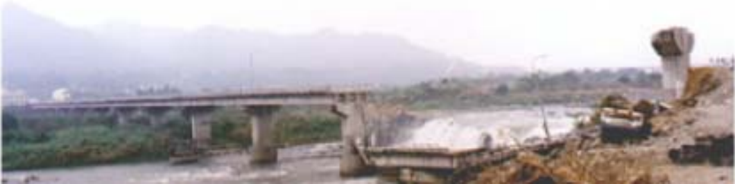
FIGURE 30.67 The Dajia River Bridge and 6-m fault scarp.
