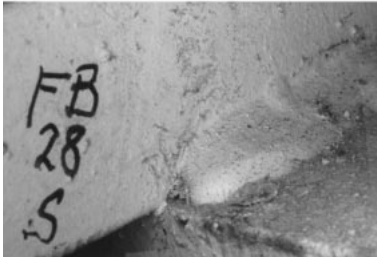
FIGURE 24.8: Fatigue crack originating from the upper weld toe of a fillet weld where the fillet weld terminates near the overlap of thick plates.
