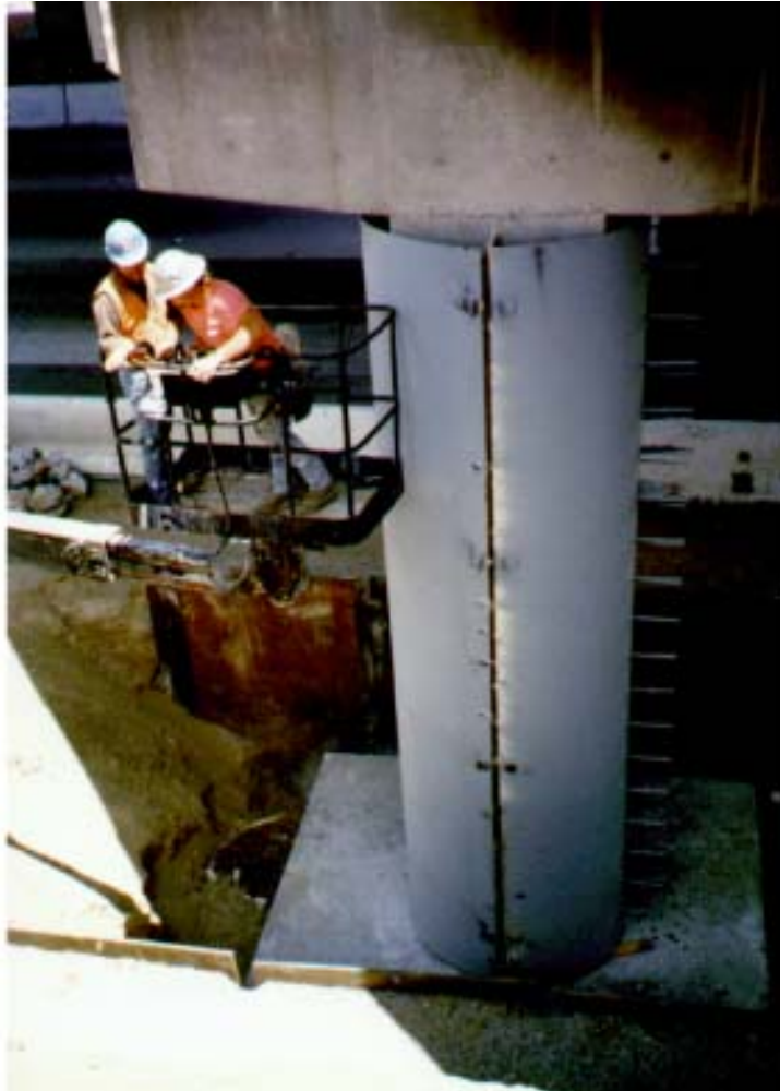
FIGURE 30.89 Steel shell being wrapped around a concrete bridge column to increase its ductility and shear strength.
