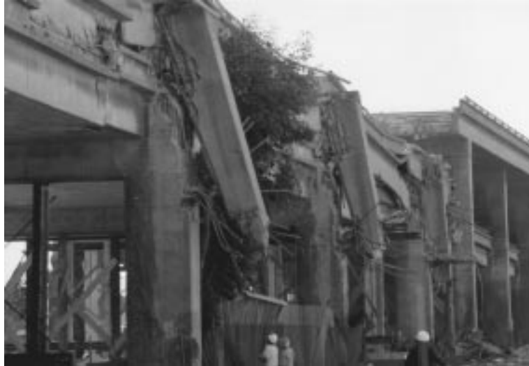
FIGURE 16.3: Collapsed Cypress Viaduct (I-880) following the 1989 Loma Prieta earthquake in California.
