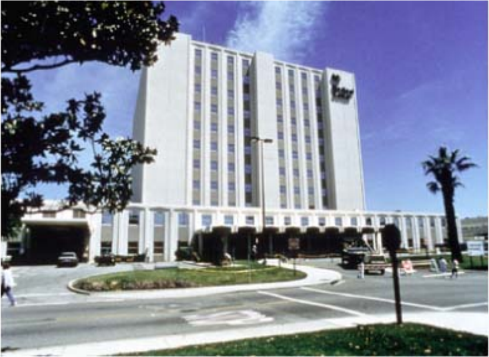
FIGURE 30.84 The existing Long Beach VA Hospital was seismically retrofitted with lead-rubber bearings. (Courtesy of Dynamic Isolation Systems, Inc.)
