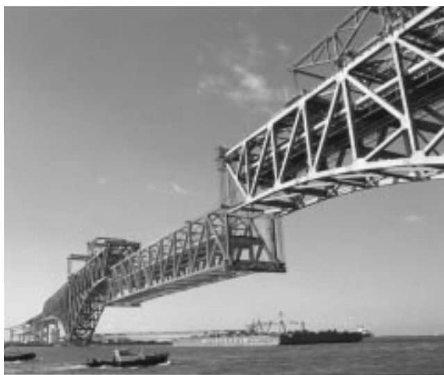
Lifting the center girder of the Minato Bridge into place.
