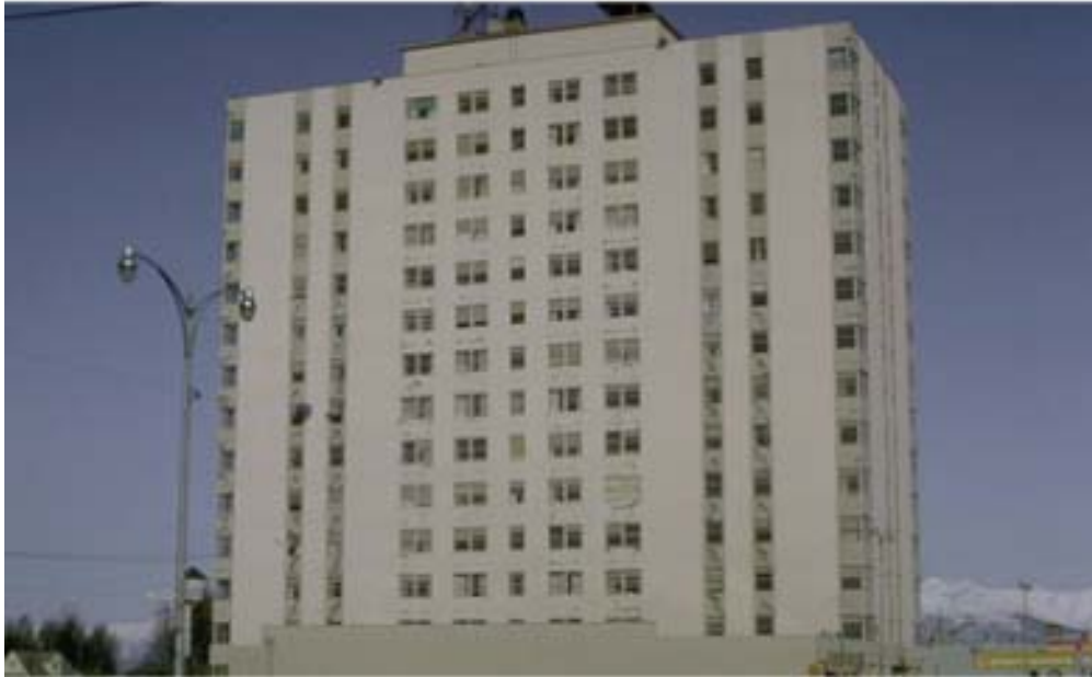
FIGURE 30.48 West elevation of Mt. McKinley Apartments after the 1964 Great Alaska earthquake. (Photograph by Karl Steinbrugge and courtesy of the Steinbrugge Collection, Earthquake Engineering Research Center, University of California, Berkeley.)
