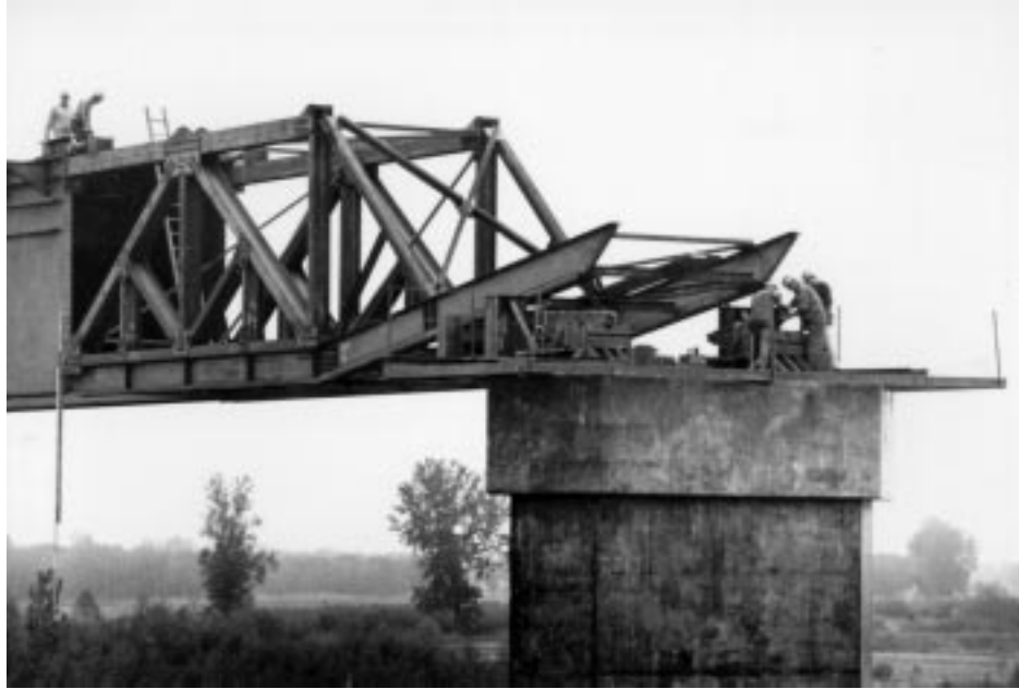
Figure 20.41b Launching nose rides up onto pier 5 skidway units, removing girder-train leading-end sag.
