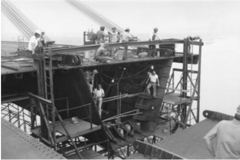
FIGURE 20.10: Luling Bridge deck steelwork erection, 1982; view looking northeast (refer to Figure 20.9) The twin box girders are 14 ft (4.3 m) deep; the deck plate is 7/16 in. (11 mm) thick. Girder section 16-east is being raised into position (lower right) and will be secured by large-pin hinge bars prior to fairing-up of joint holes and permanent bolting. Temporary erection stays are jumped forward as girder erection progresses.
