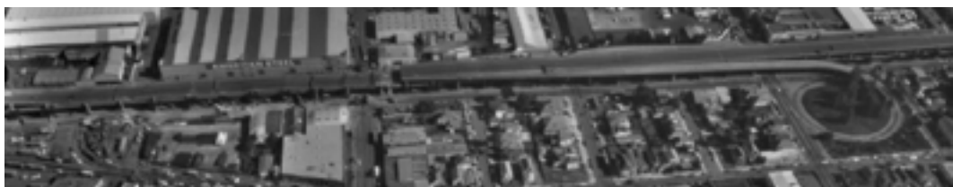
FIGURE 30.29 Aerial view of Cypress Street Viaduct showing collapse at north end (left) where the structure crossed over Bay mud, while the southern part (right), supported by dense sand, remained standing.
