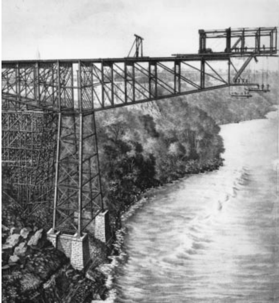
FIGURE 20.17: Niagara River railway cantilever truss bridge, near Niagara Falls, New York 1883. Massive wood erection traveler constructed side span on falsework, then cantilevered half of main span to midspan. Erection of other half of bridge was similar. First modern-type cantilever bridge, with 470-ft (143-m) clear main span having a 120-ft (37-m) center suspended span.
