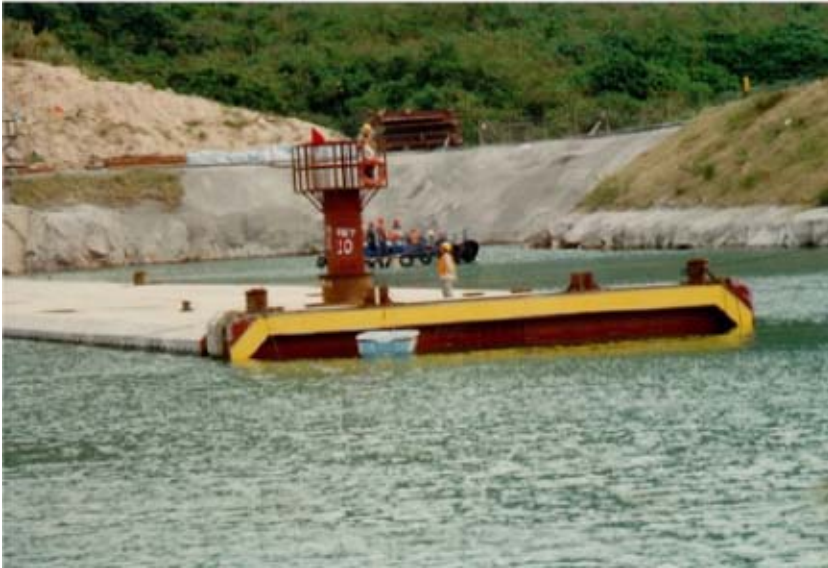
FIGURE 15B.2 Floating element: airport rail tunnel, Hong Kong. (© Christian Ingerslev.)
