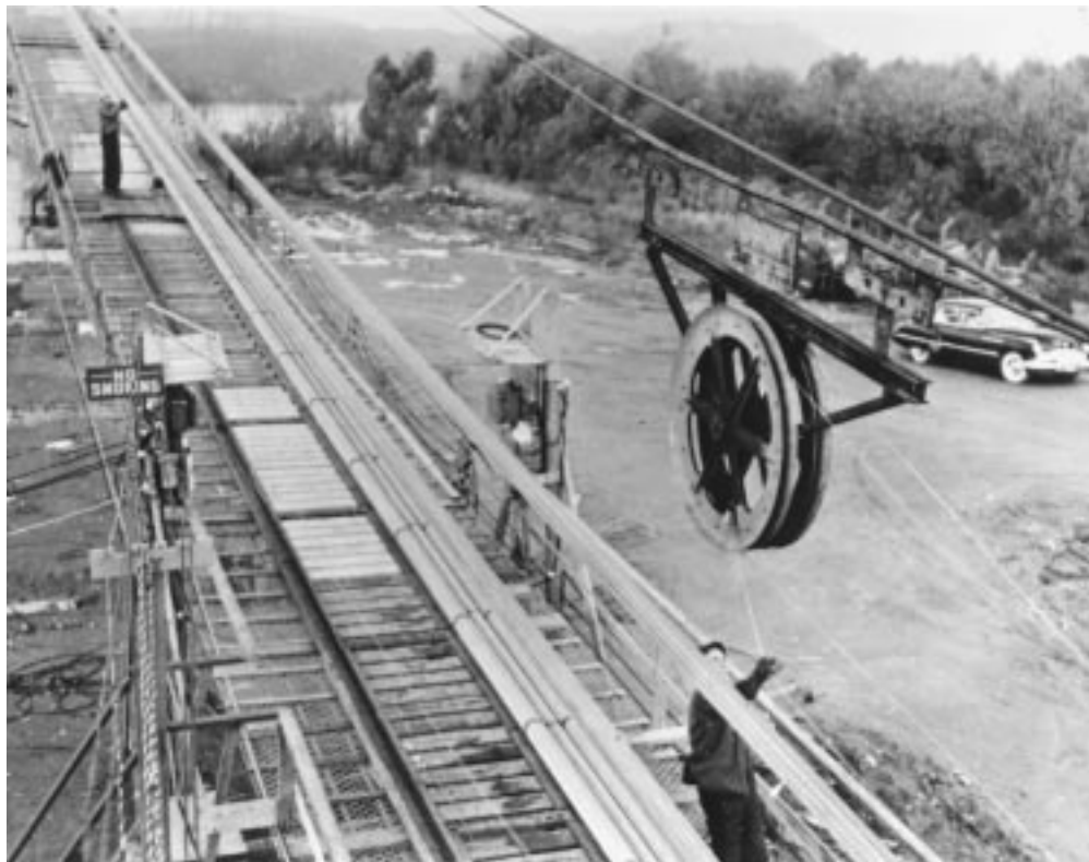
Figure 20.25a Tramway starts across from east anchorage carrying two wire loops. Three 460-wire strands have been spun, with two more under construction. Tramway spinning wheels pull wire loops across the three spans from east anchorage to west anchorage. Suspended footbridges provide access to cables. Spinning goes on 24 hours per day.
