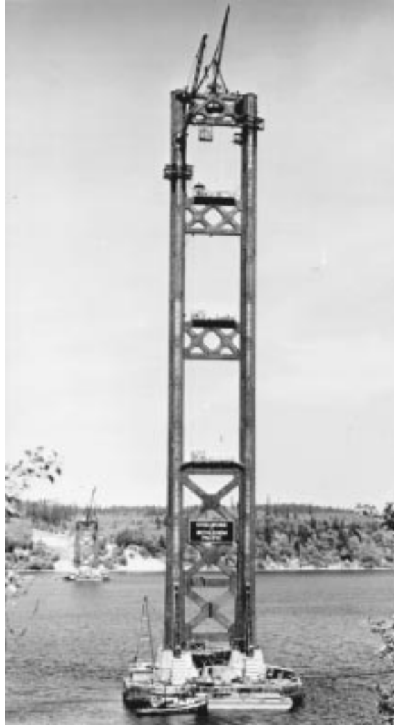
FIGURE 20.24: Tower erection, second Tacoma Narrows Bridge, Washington, 1949. This bridge replaced first Tacoma Narrows bridge, which blew down in a 40-mph (18-m/sec) wind in 1940. The tower legs are 60 ft (18 m) on centers and 462 ft (141 m) high. The creeper traveler is shown erecting the west tower, in background. On the east tower, the creeper erected a Chicago boom at the top of the south leg; this boom dismantled the creeper, then erected the tower-top bracing and a stiffleg derrick, which proceeded to dismantle the Chicago boom. The tower manhoist can be seen at the second-from-topmost landing platform. Riveting cages are approaching the top of the tower. Note tower-base erection kneebraces, required to ensure tower stability in free-standing condition (see Figure 20.27).
