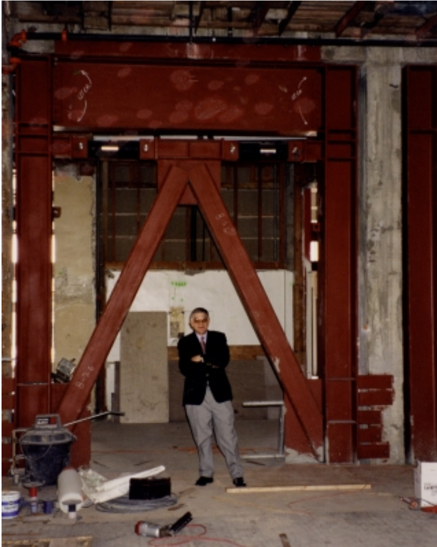
FIGURE 30.83 The steel frames included fluid viscous dampers to reduce story drift. (Courtesy of Marr-Shaffer & Miyamoto, Structural Engineers.)
