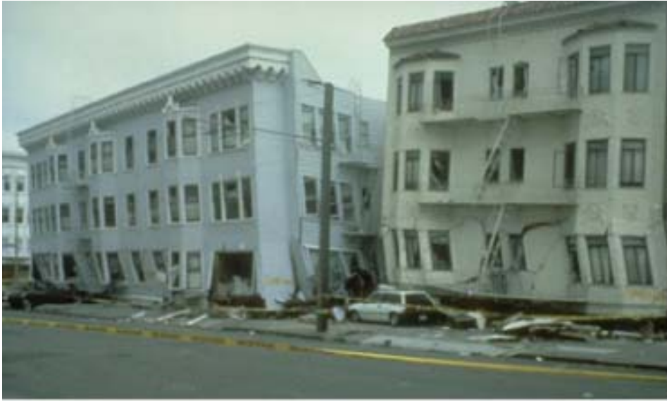
FIGURE 30.37 Soft-story collapse in San Francisco during the 1989 Loma Prieta earthquake. (Courtesy of the U.S. Geological Service [10].)
