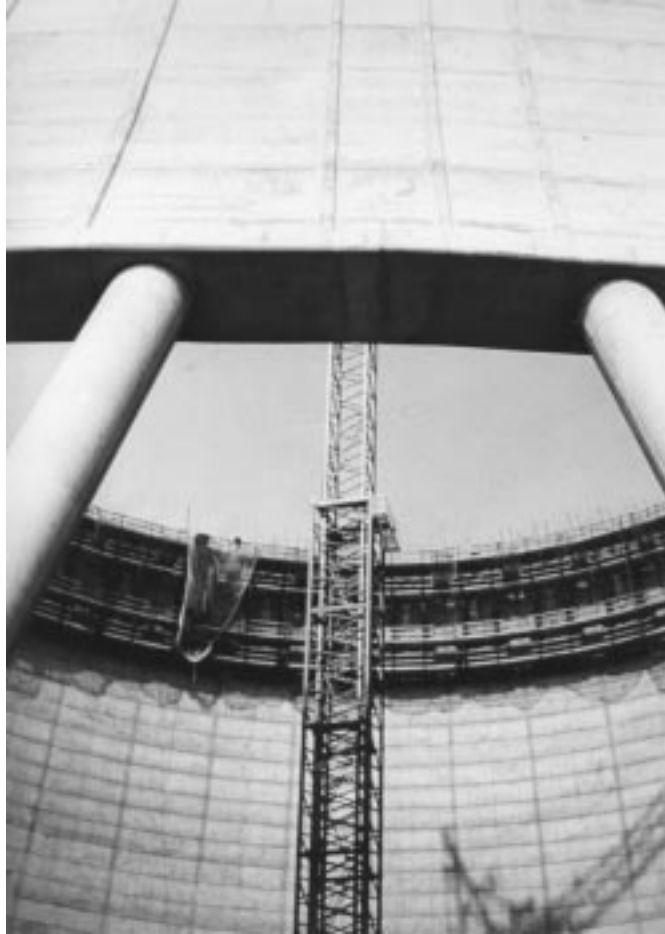
FIGURE 14.6: Climbing construction of the shell.
