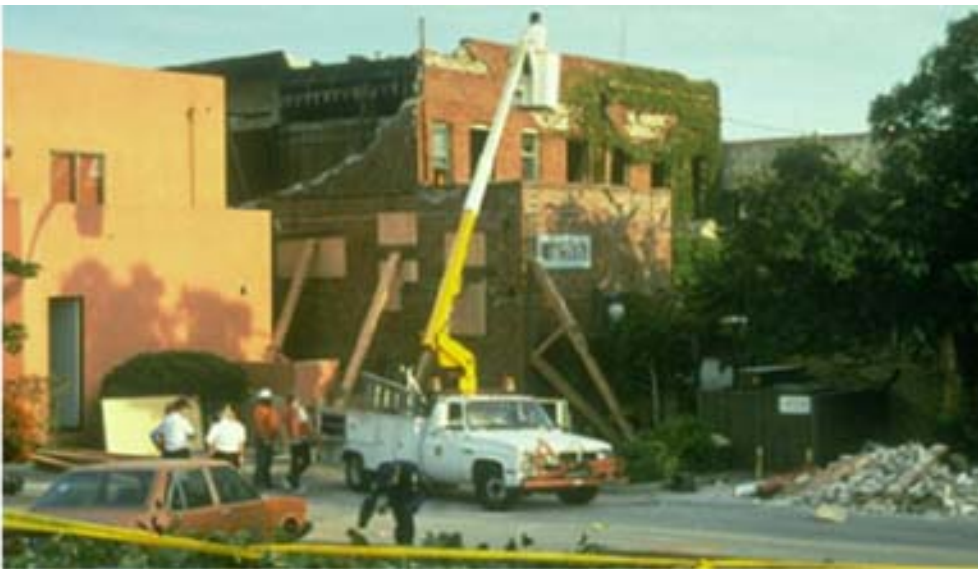
FIGURE 30.61 Rear view of damaged unreinforced masonry (URM) building facing Pacific Garden Mall, Santa Cruz Area, CA. (Photograph by James R. Blacklock, Loma Prieta Collection, Earthquake Engineering Research Center, University of California, Berkeley.)
