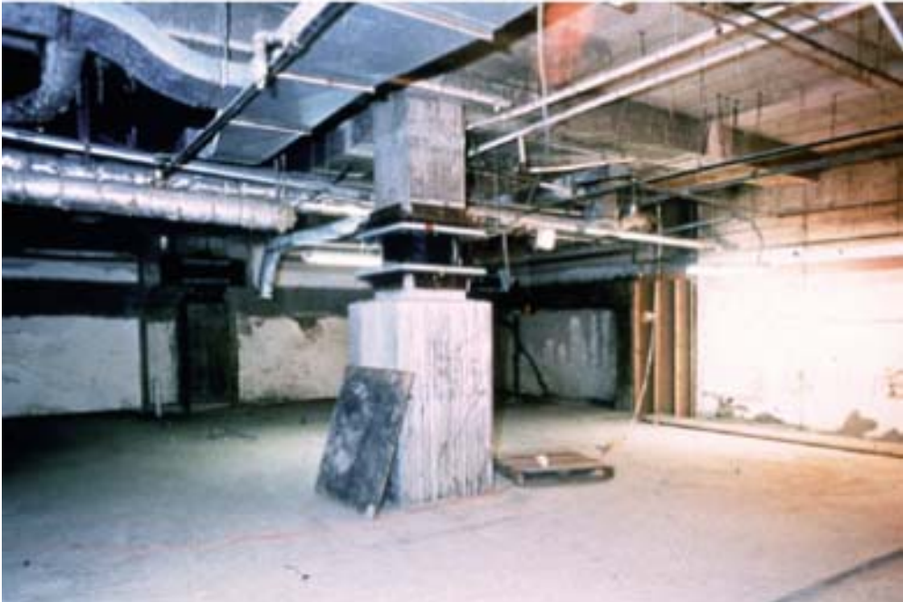
FIGURE 30.85 Concrete columns at Long Beach VA Hospital that were cut at mid-height and installed with lead-rubber isolation devices. (Courtesy of Dynamic Isolation Systems, Inc.)
