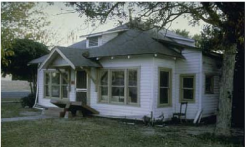
FIGURE 30.34 House that fell from its foundation during the 1971 San Fernando earthquake. (Courtesy of Steinbrugge Collection, Earthquake Engineering Research Center, University of California, Berkeley.)
