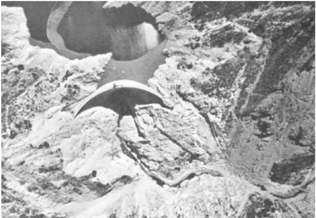
FIGURE 30.20 Landslides at Pacoima Dam following the 1971 San Fernando earthquake. (Courtesy of Steinbrugge Collection, Earthquake Engineering Research Center, University of California, Berkeley.)
