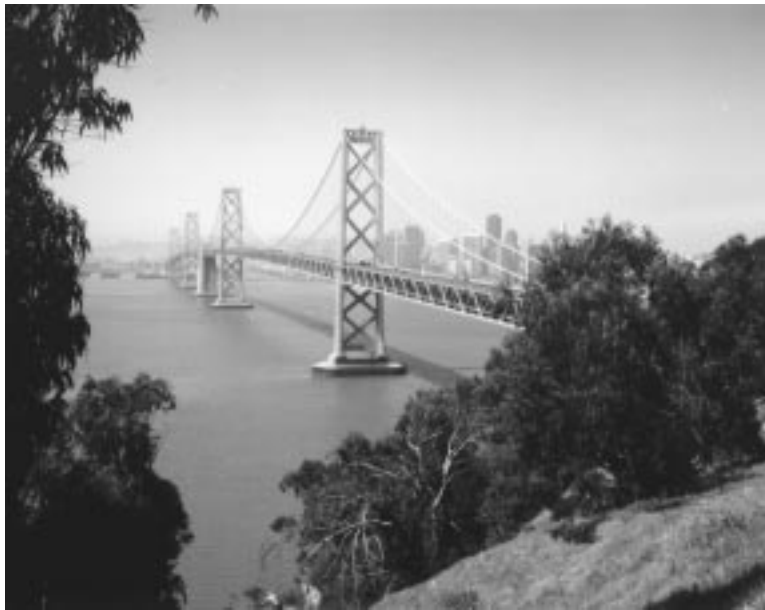
(a) West crossing spans.
